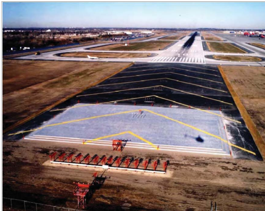
FIG 2-3-42 Engineered Materials Arresting System (EMAS)
