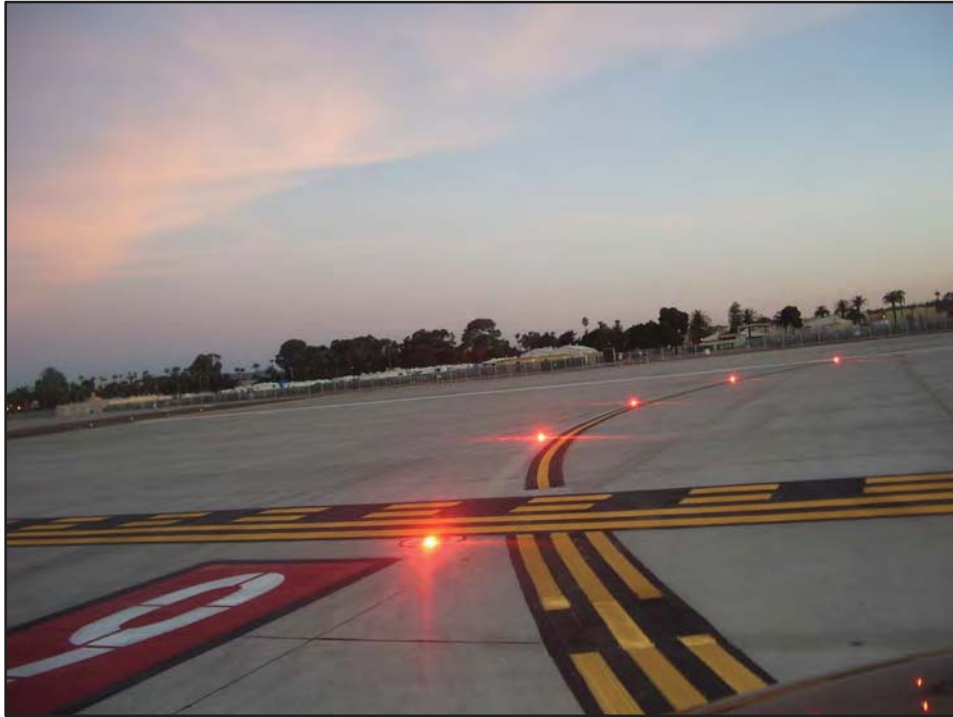
FIG 2-1-12 Runway Entrance Lights
